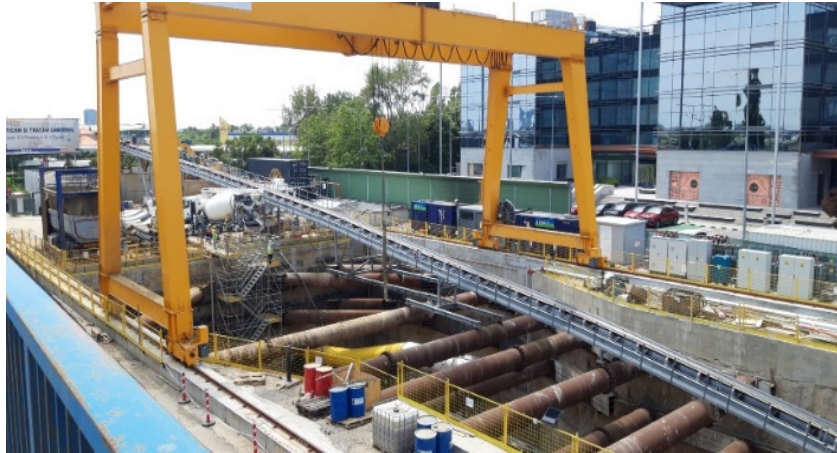
Figure 3: Portal crane – M6 metro line construction site, Bucharest
