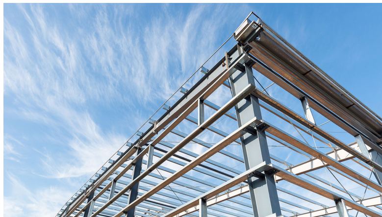
Figure 3: Modular and prefabricated steel systems facilitating reuse. [F3]
